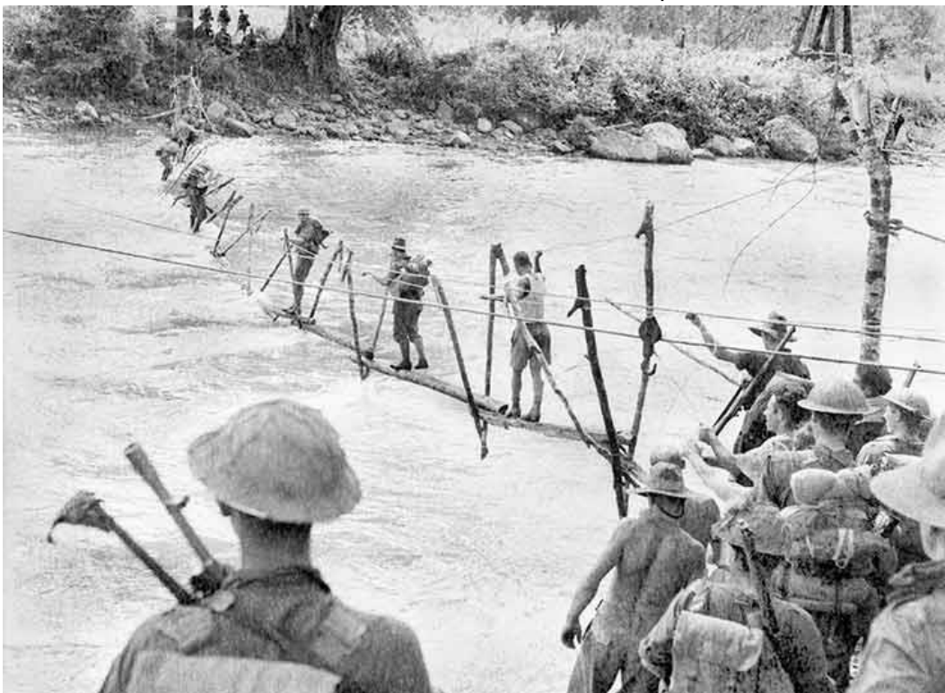
Kumusi River Bridge.
